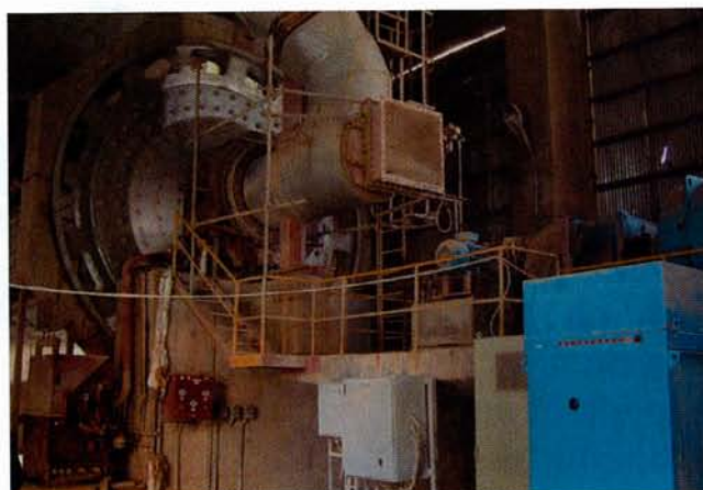
1 Ball mill with oil cooled starter
