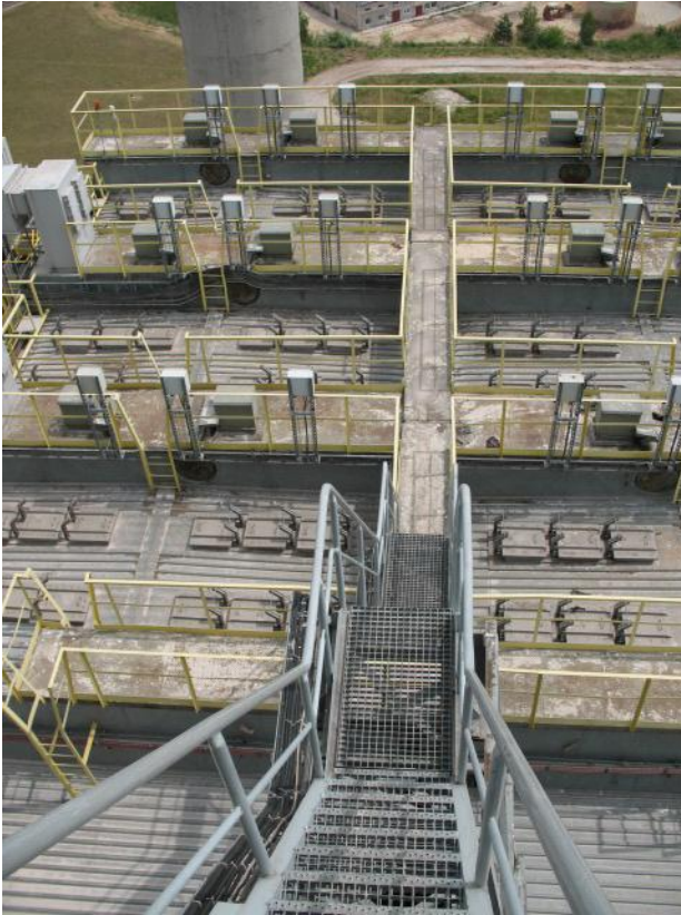
ESP top view before retrofit
