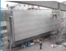
On site erection of the new bag filter.
