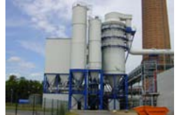
Flue-gas dust removal in the waste disposal industry
