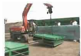
4. Assembly on site of the complete filter head
