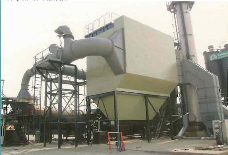
1. Complete new installation.
