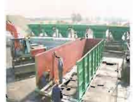
2. Conversion of Wibau filter
