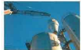
Erection and commissioning, service and repair of gas-scrubbing plants.
