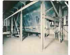
Sorption installation after a sewage incinerator for separation of off-gas components according to regulation 17 BimSchV.
