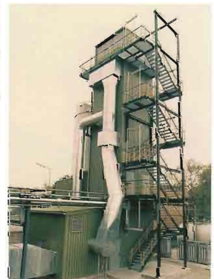
Dry sorption installation after a special-waste incinerator rotary kiln.
