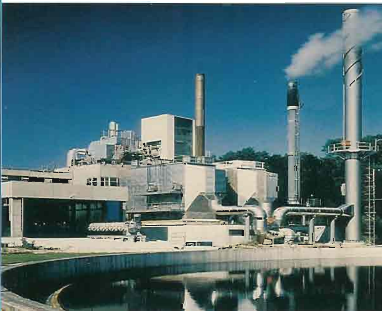
Dry sorption installation after a special-waste incinerator rotary kiln.
