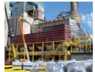
quired in advance. A total of approx. 200 t of steelwork was assembled for the supporting structure, maintenance platform and railings, and approx. 180 t of ducting with diameters of 3.00 m and 4.50 m was installed.
