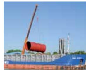
900 t of material were shipped across the Baltic Sea to Gotland. The retrofit and assembly work took place from May to October 2009. With dimensions of 33 m length, 15 m width and 22 m height, extensive construction work was re-
