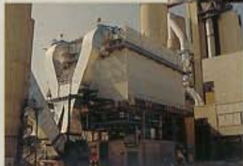
Erection of a filter unit for kiln raw meal mill and quencher
