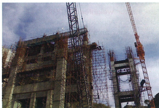
1 Ambuja Cement Limited construction site
