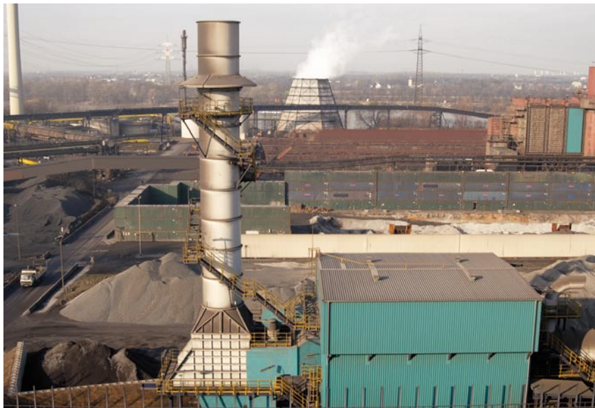
Figure 1. Filter No. 5 of the HKM steel works
