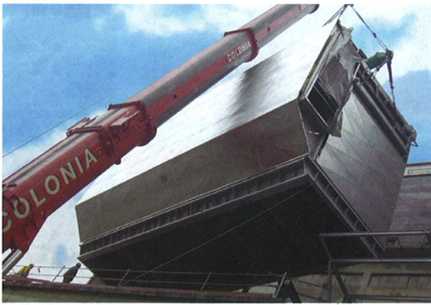
Figure 5. Installation of pre-assembled filter housing (2007).
