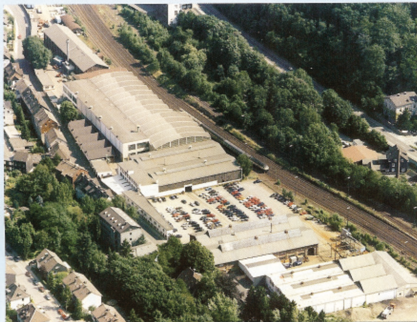
Aerial photo of the production facility at the headquarter of Intensiv Filter in Velbert-Langenberg
